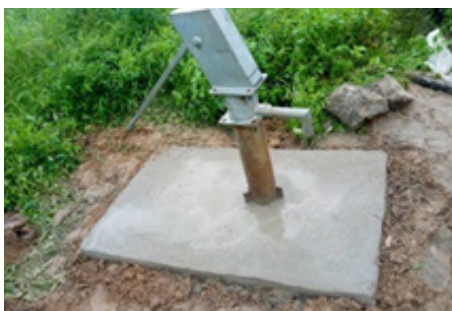
Rehabilitation of the school water system (Borehole)
