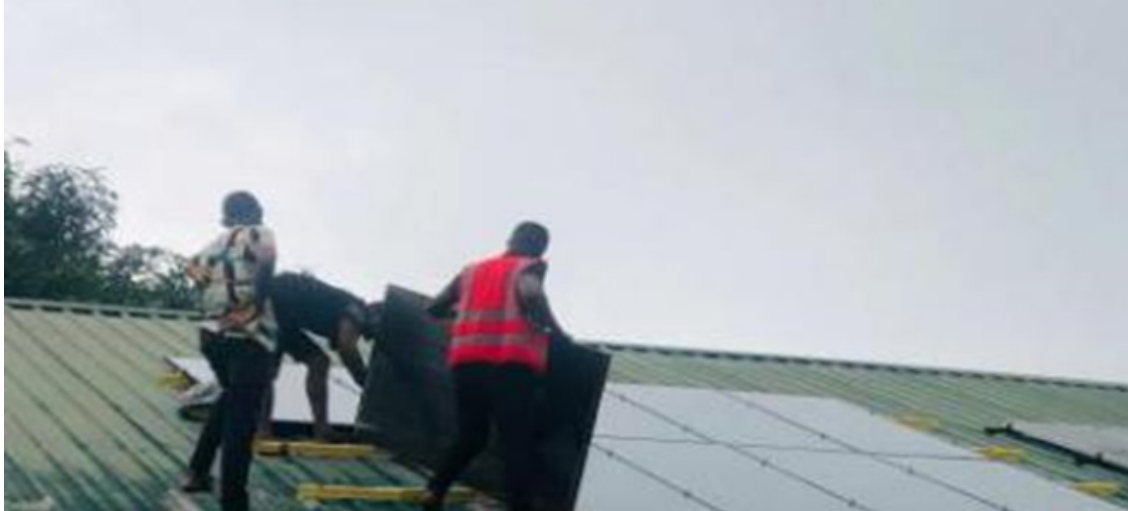
Vendors installing solar panels at PHC West Itiam
